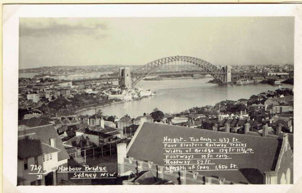
Harbour Bridge, Sydney, N.S.W. (Anon)
