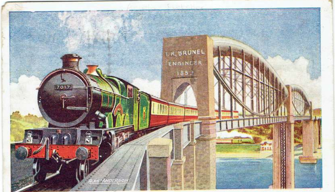
BRITISH RAILWAYS. WESTERN REGION. A Cornish express crossing the famous Royal Albert Bridge, Saltash, which spans the Tamar estuary to link Devon and Cornwall. It was Brunel's final and greatest engineering feat. Each of the two main spans is 455 ft. in length with long approach arches.
